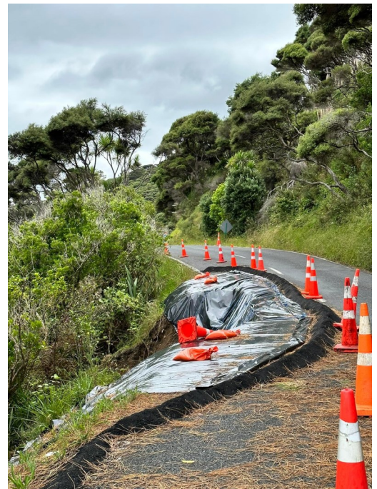
Above: Example of polythene over slip face, combined with bunding treatment.
